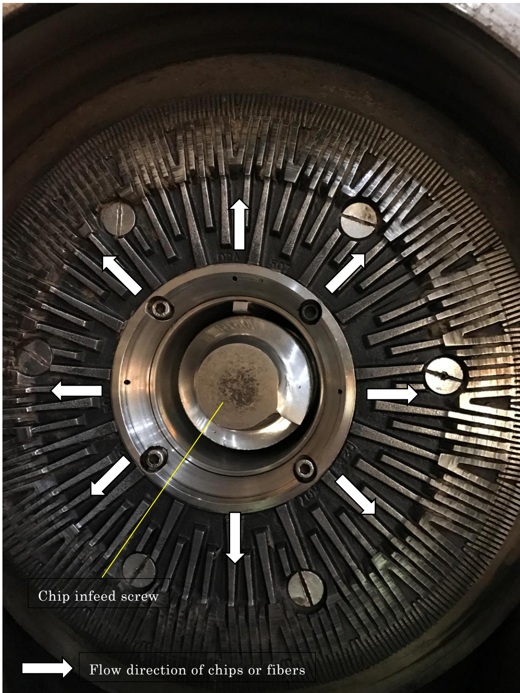
Fig.4-5 Inside the refiner (Stator side).
